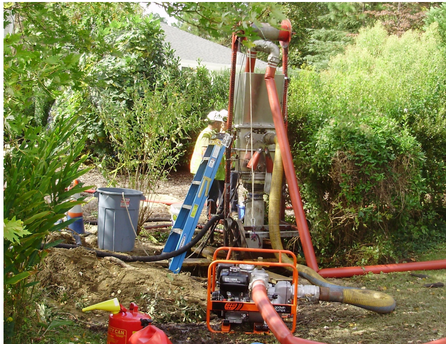
Sewer Slip Lining Work In Process
