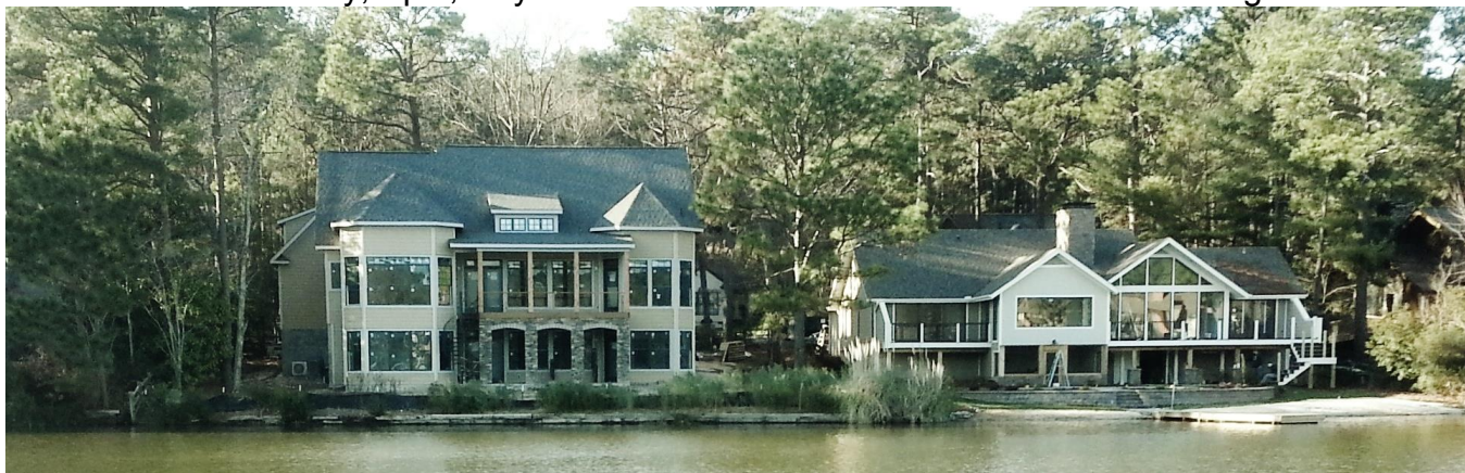
New Construction & Major Rehab on the Lake
